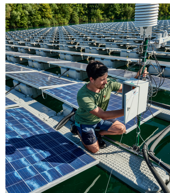
Installation of measuring devices (left) and floating PV system near Renchen/Baden (right). © Jan Oelker
